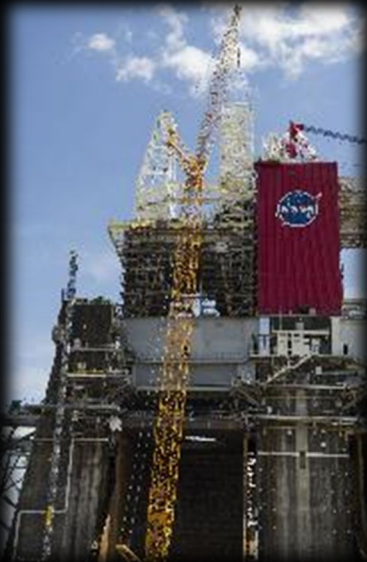
B-2 Test Stand modifications for SLS Core Stage Testing
