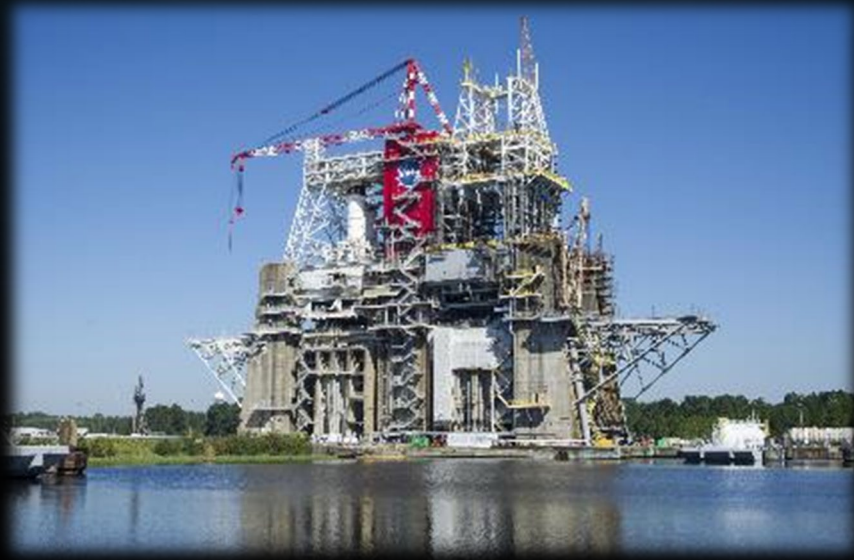
B-2 Test Stand modifications for SLS Core Stage Testing
