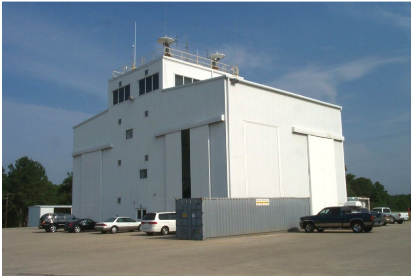
ACES-01 was assembled and tested in this NSBF hanger
