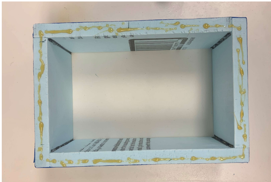
Figure 10: Apply glue to the bottom edge of the outside wall piece
