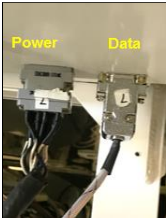
Fig. 10 Connection of power and data communication cables of HASP with the payload (#7).
