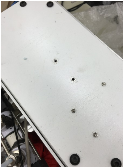
Figure 30: Top view of the system showing missing screws
