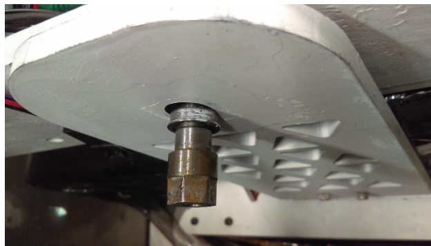
Figure 36: Bearing Knocked Out of Place
