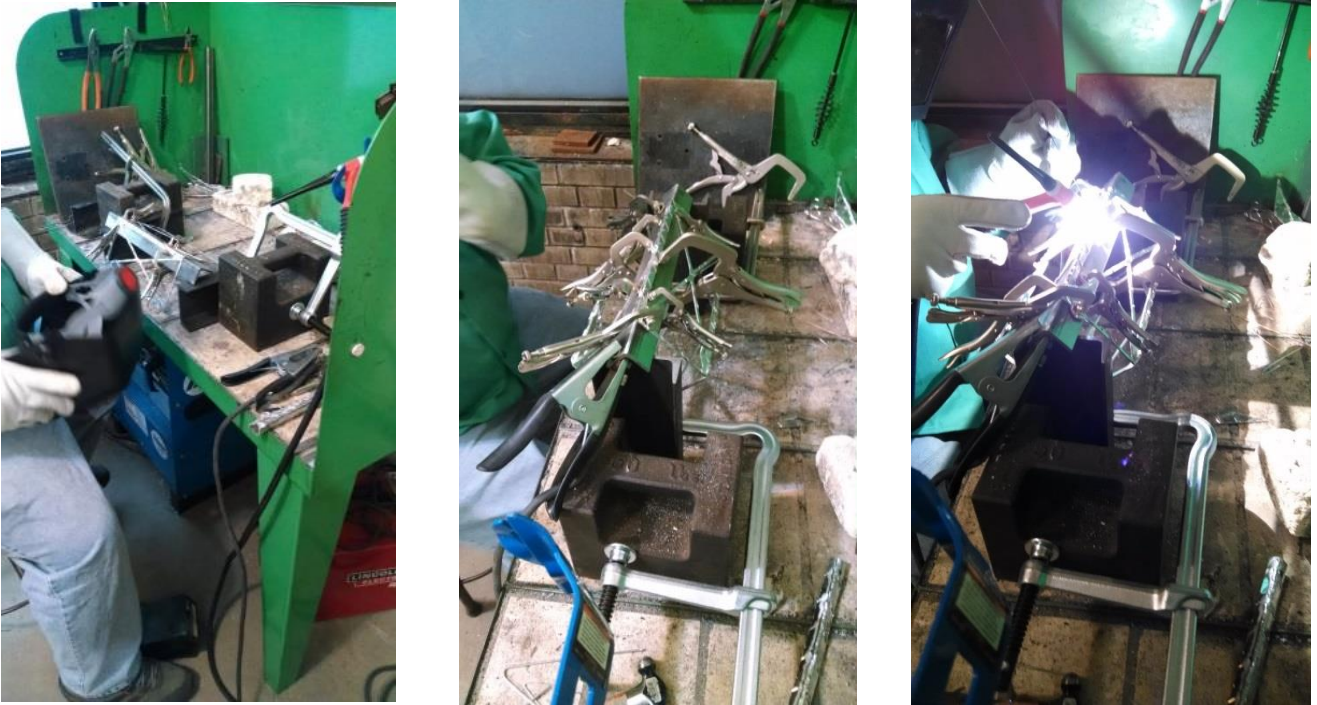
Fig 11. Welding of the Aluminum Frame
