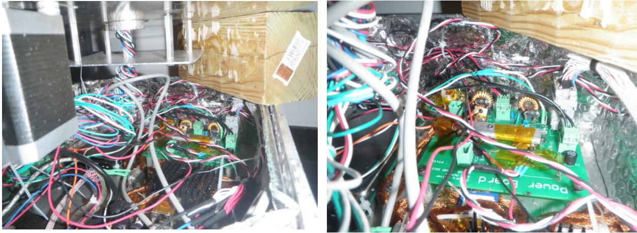
Figure 14: Wires Became Tangled and Disconnected as Platform Rotated
